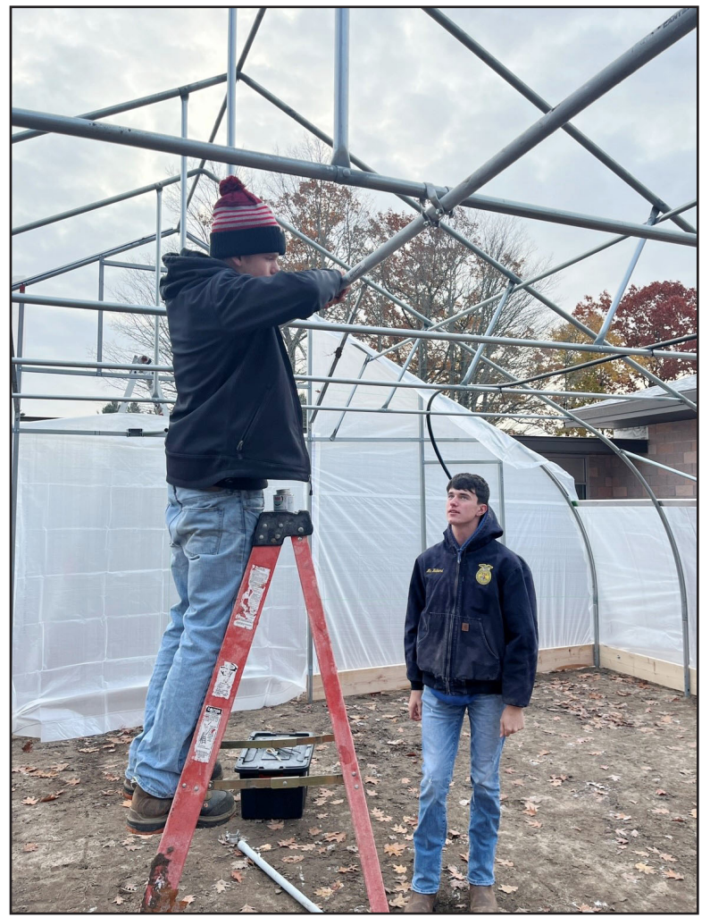
Students Gavin Dellar (left) and Daniel June (right) assemble the hoop house for the agri-science aquaponics program. Courtesy photo.
