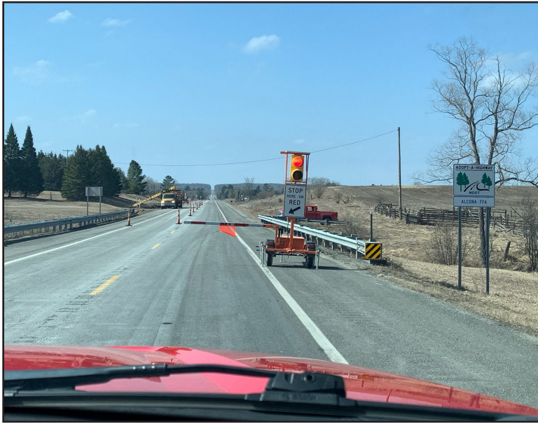
The Alcona County Road Commission will be using two new Automated Flagger Assistance Devices during road construction projects. Courtesy photo.
