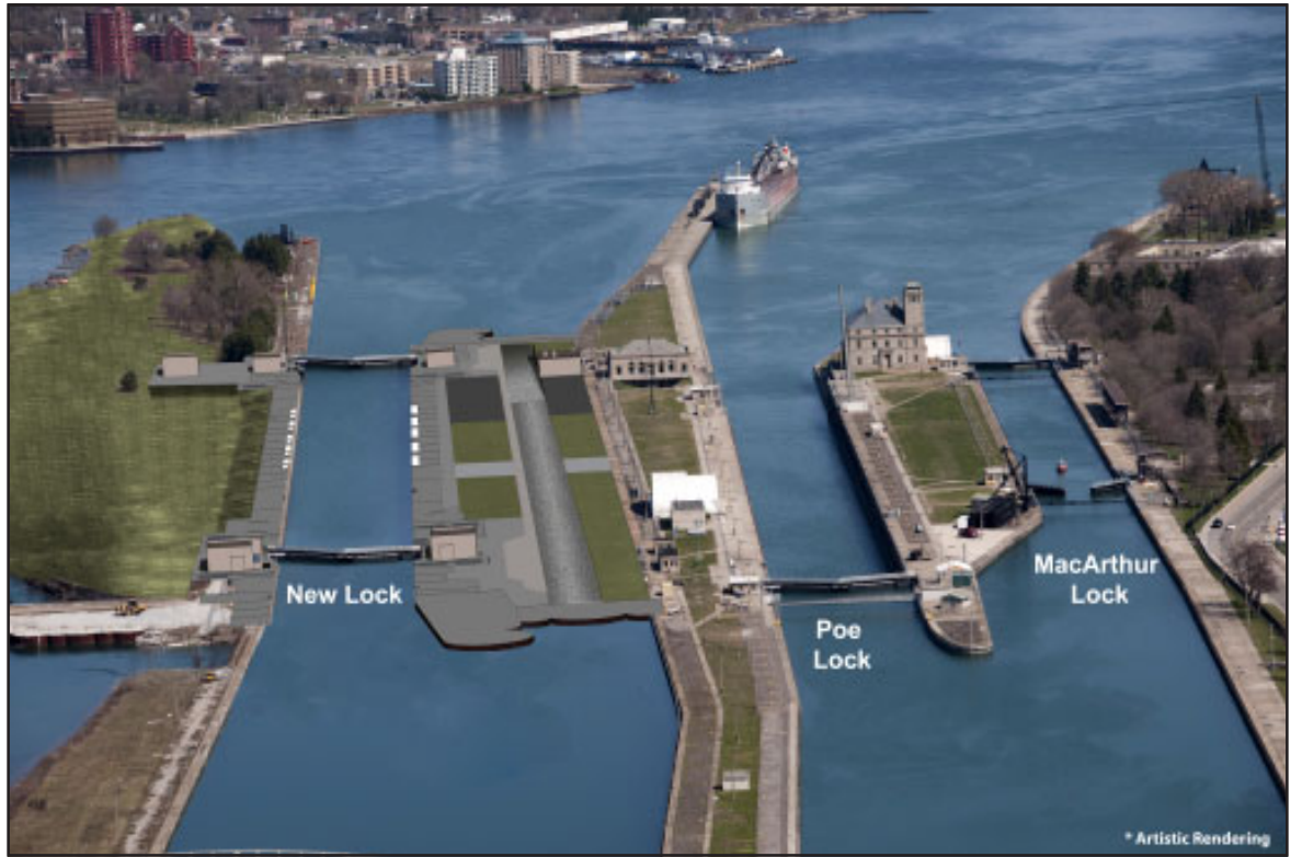
This image is an artist rendition that illustrates what it might look like if a second Poe-sized lock replaced two of the older locks (left portion of the photo). The Poe Lock, opened in 1969, was the last lock built in the Soo Locks system, the only passage between Lake Superior and the lower lakes. (Second Poe-Sized Lock far left, Poe Lock center, MacArthur Lock far right.) Courtesy of U.S. Army Corps of Engineers
