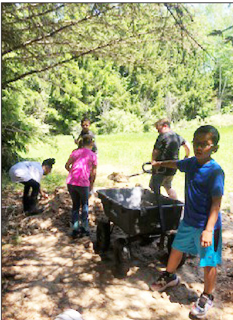
Third-grade students become erosion engineers by tackling a problem with a holding pond that was washing out part of the trail on the school district's 42-acre placed-based education area. The project encompassed much of their school year and incorporated science, technology, engineering and math plus reading, writing and English lessons. Along with their classmates, (from left) Isabell Liebler, Geri Kirk, Taylor Laube, Emma Hechlick and Noah Lafeldt contributed physical labor to the project as well. Courtesy photo.
