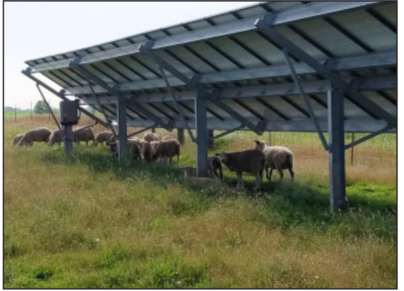
Sheep graze under the shade of solar panels in Lenawee County, an example of agrivoltaics. Photo courtesy of Charles Gould/CNS.
