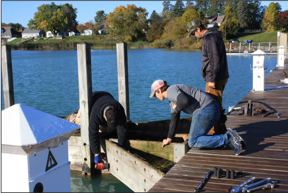
Workers from Water Street Adventures (from left), Allan Griffin, Noah Grenke and Justin Rau removing a finger pier dock. Photos by Mary Weber.
