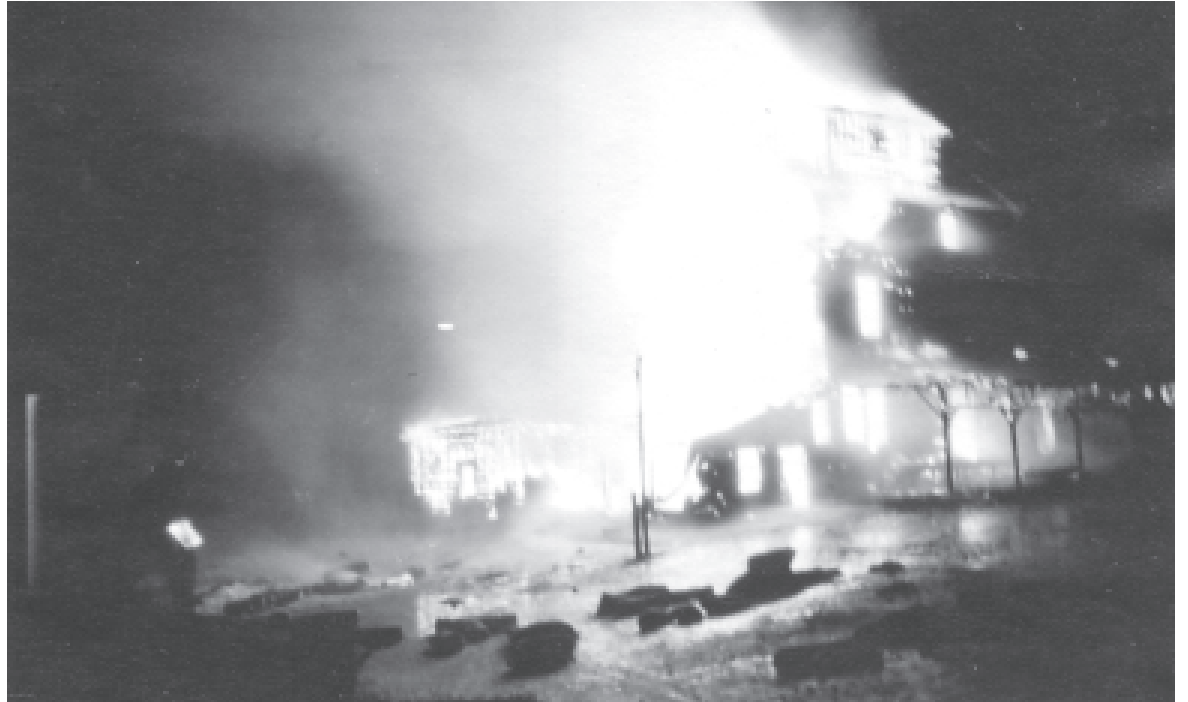
Lincoln Elevator fire Friday, Jan. 27, 1922.
