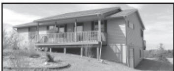
Harrisville-Three bedroom 2 1/2 bathroom raise ranch with a covered front porch, over a full walk out basement. 19-0029 $279,900
