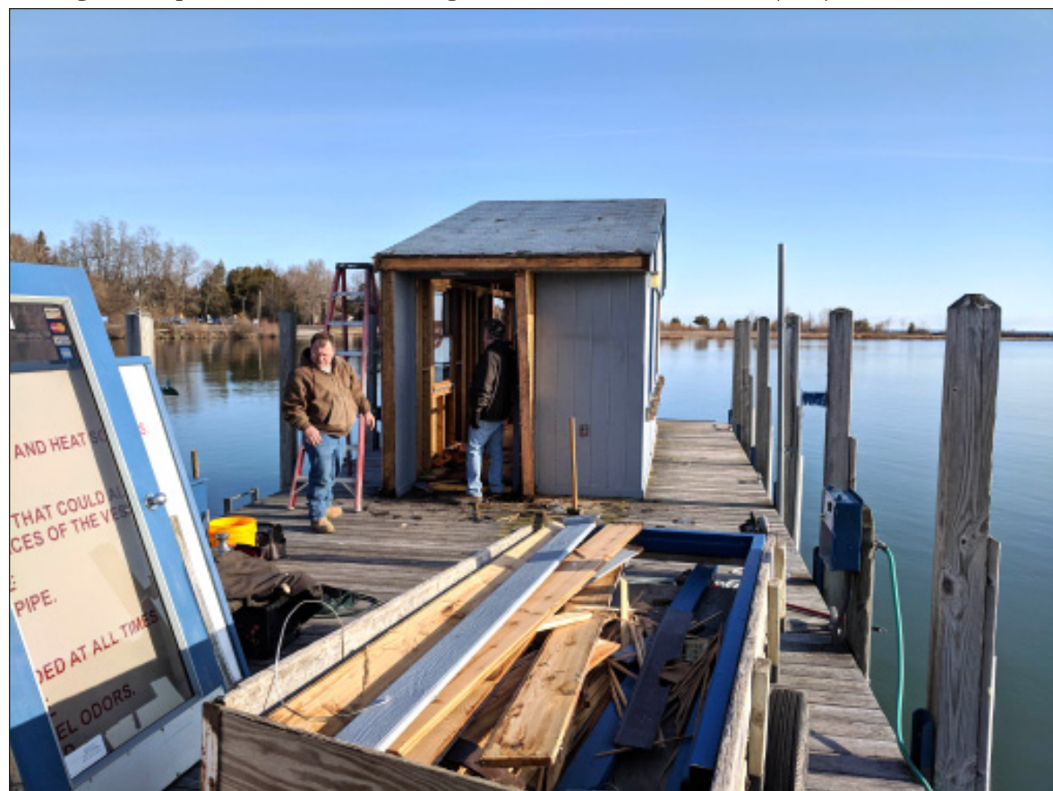
Workers dismantle the structure. Photo courtesy of Jim Ferguson.
