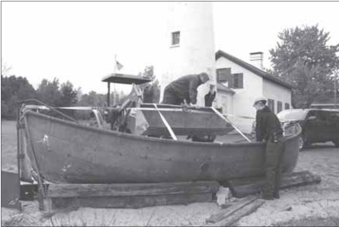
A long standing goal of the Alcona Historical Society was achieved recently when the Reames boat at the Sturgeon Point Lighthouse was moved to a safer location on a concrete pad with a structurally sound cradle. The life boat from an unknown ship was donated to the group by the Reames family after finding it covered with leaves and debris in their woods around the late 1990s. It was built by David Kahnweiler and Sons April 4, 1906 in New York. (from left) Eric Ostrander, manager of the Harrisville State Park, Michael Signorello and Allan Baldwin (not in photo) lifted the Reames from its deteriorating cradle and carried it to the new secure station. Photo by Mary Weber.
