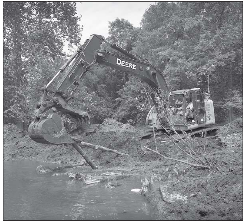
The logs, positioned perpendicular to the bank, are known as "toe wood."
