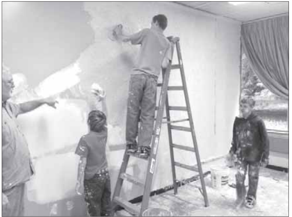
Alcona students Daniel Fulsher, Sammy Hendrickson and Dustin Grabow, under the supervision of special education teacher Rick Sedgwick, texture a wall at Alcona High School. They were involved in patching holes, applying the texture material, and troweling the texture into a finished product. According to Sedgwick, this is "just another facet of our Vocational Education Initiative at Alcona High School."
