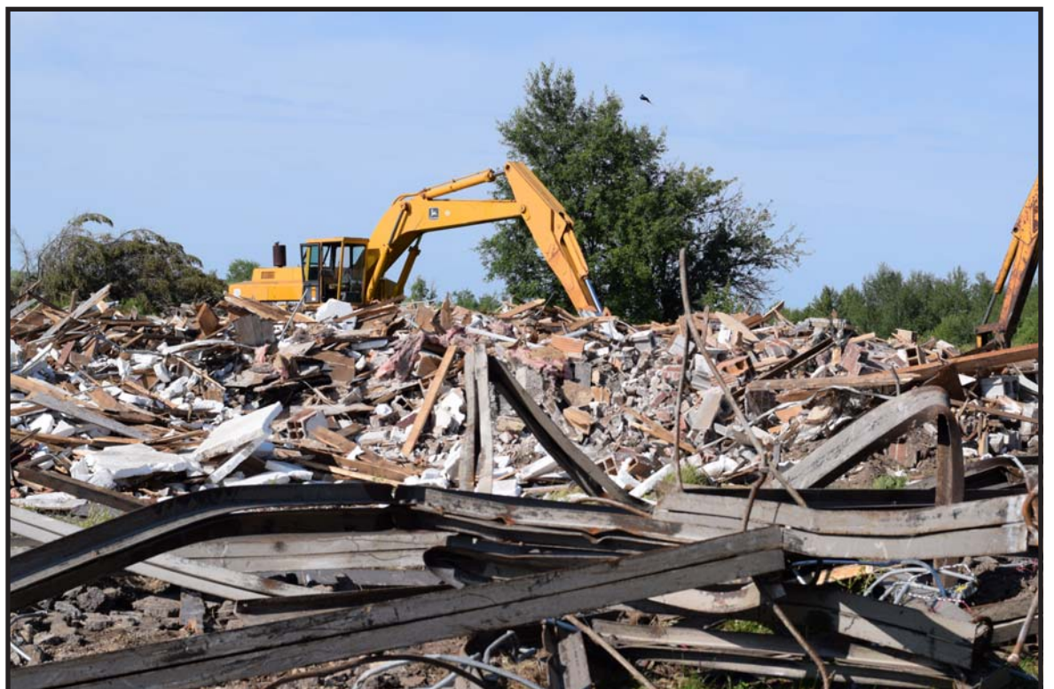
The hall was constructed prior to the use of asbestos and lead paint in building material. Photo by Kirk Walton.
