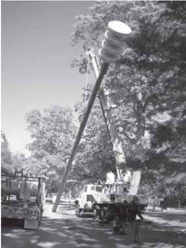
An emergency siren is installed at Muskallonge Lake State Park as part of the StormReady program. Sirens have been used at the park to warn campers of wind storms and other severe weather approaching off Lake Superior. Photo courtesy of Michigan DNR.
