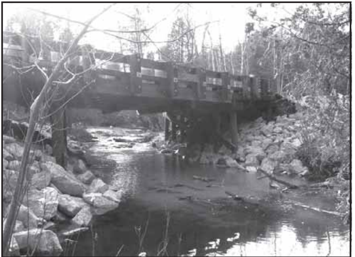
The new bridge on Sucker Creek Road will keep sediment from being deposited into the stream and keep the road from being flooded -- a familiar occurrence when the twin culverts (right) were in place. Courtesy photos.
