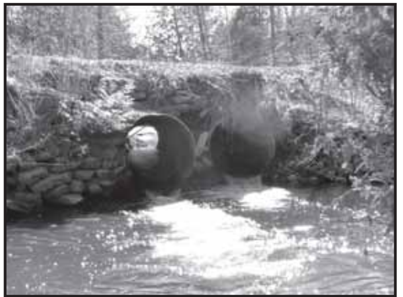
The new bridge on Sucker Creek Road will keep sediment from being deposited into the stream and keep the road from being flooded -- a familiar occurrence when the twin culverts (right) were in place. Courtesy photos.
