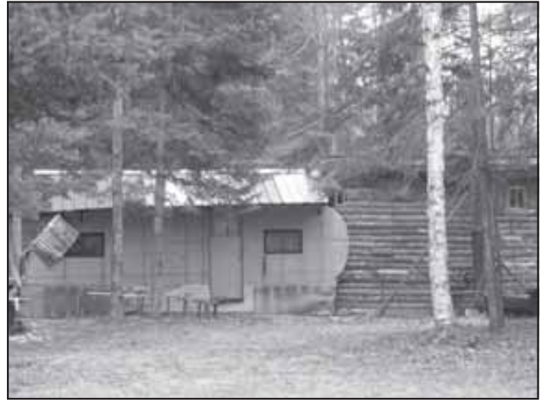
An encroachment in Montmorency County, showing a garage structure that is partially on public land and a trailer (to the left) that is entirely on public land. (The property line runs approximately through the door handle of the larger entry door on the left of the structure.)
