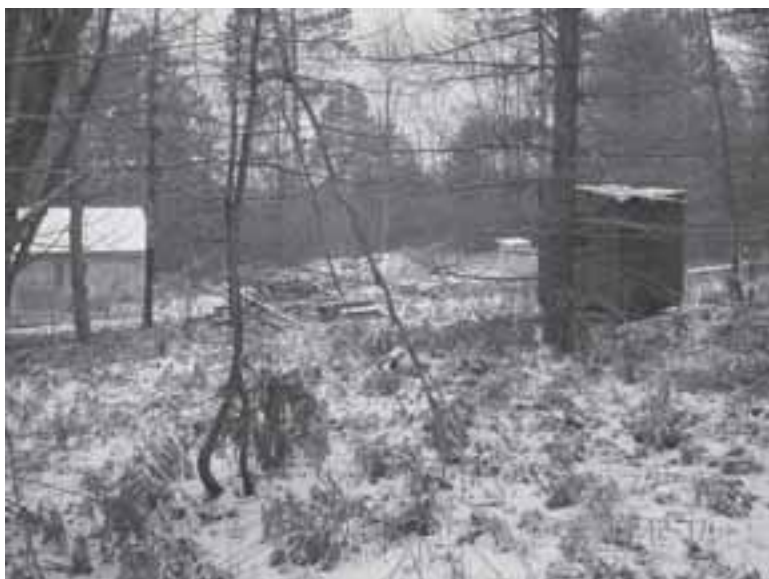
A historical encroachment in Presque Isle County, showing two smaller structures on the right that are entirely on public land and a larger cabin (on the left) that is partially on public land. (The property line is at the left edge of the photo.) Photos courtesy of Michigan DNR.
