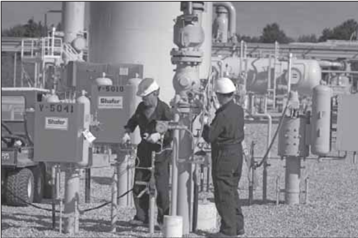
Workers lubricate the valves at an underground natural gas storage well. Almost 40,000 acres of state land is used for underground natural gas storage. Some 6,000 acres of storage was added in 2007. Photos by David Kenyon, Michigan DNRE.
