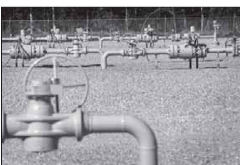
Each wellhead represents a separate underground natural gas storage well.
